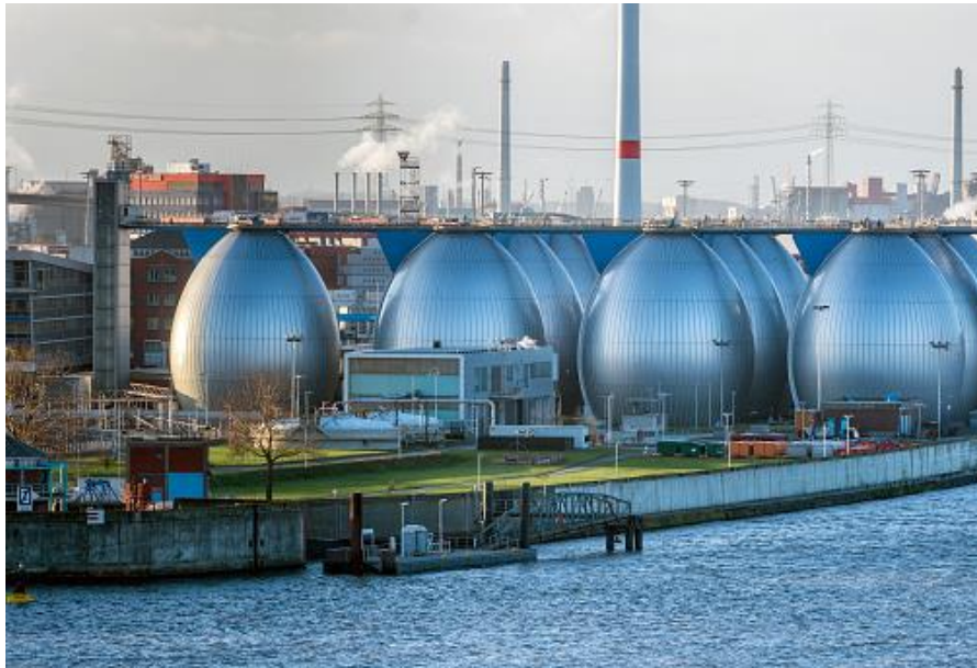
Desalination by distillation in Hamburg Germany
