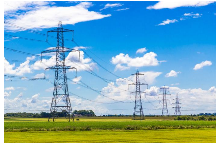
Pylons carry overhead power cables
